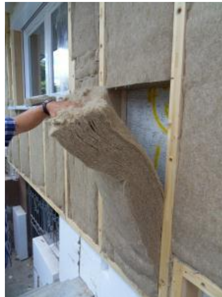
AW, Fassadensystem TH WOOD U = 0.19 \text{ W/m}^2\text{K}
